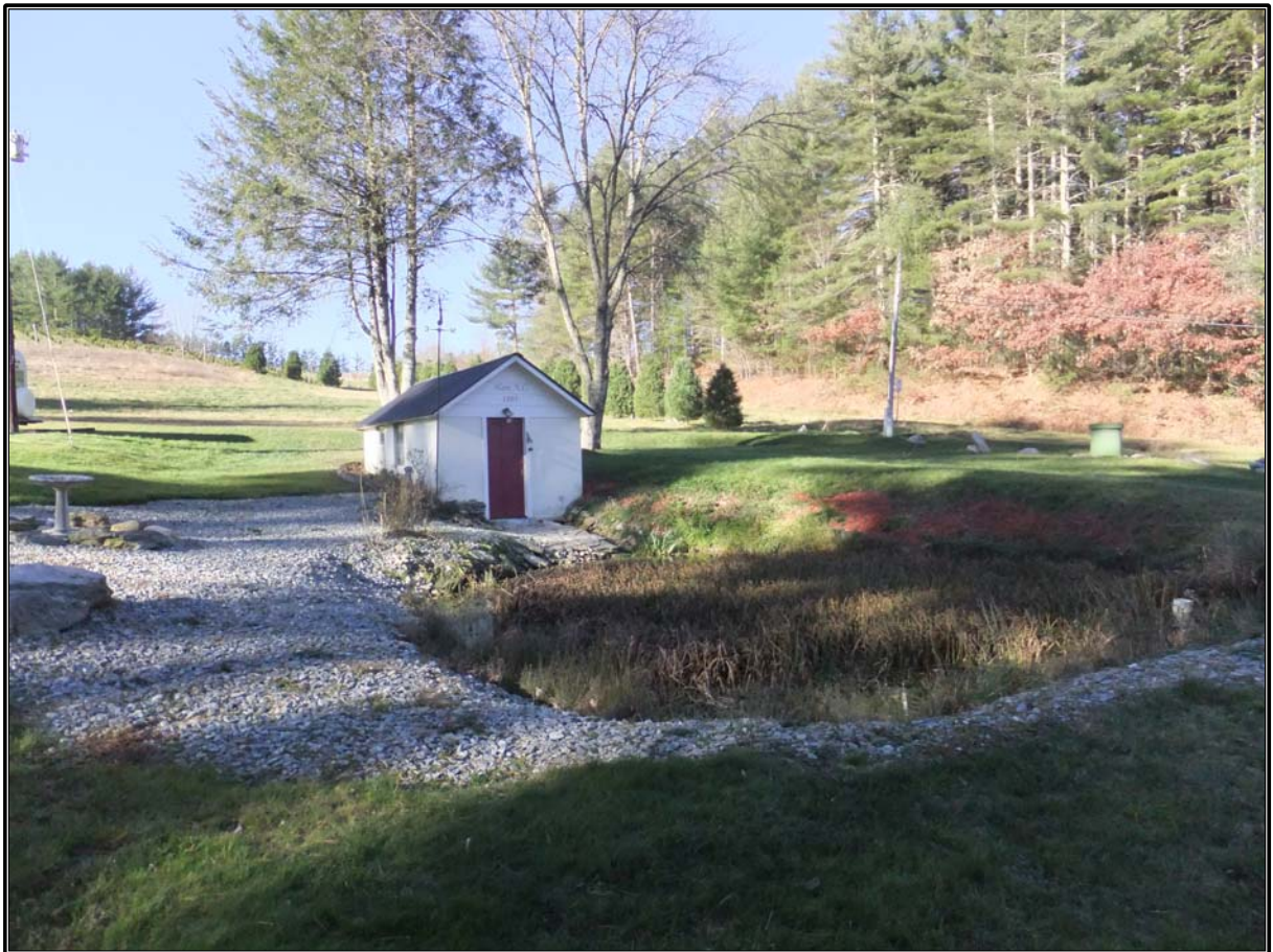
Figure 26. R.L. Hendrix House (AL 198): Southwesterly view of springhouse.
