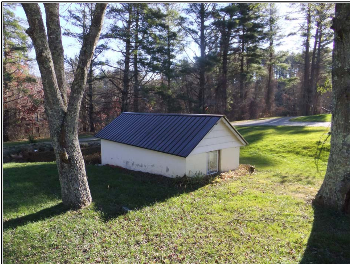
Figure 27. R.L. Hendrix House (AL 198): Rear of springhouse.
