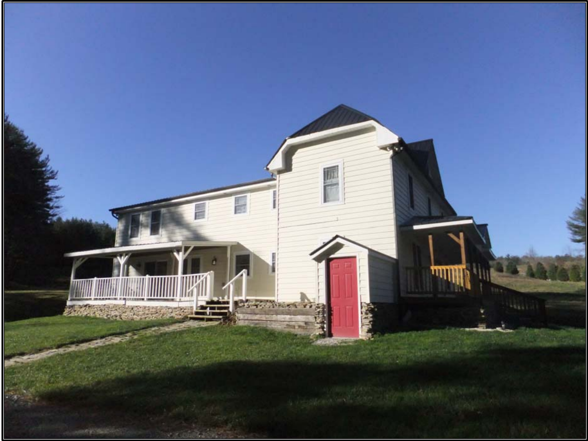
Figure 8. R.L. Hendrix House (AL 198): Southwesterly view of east elevation and rear additions.
