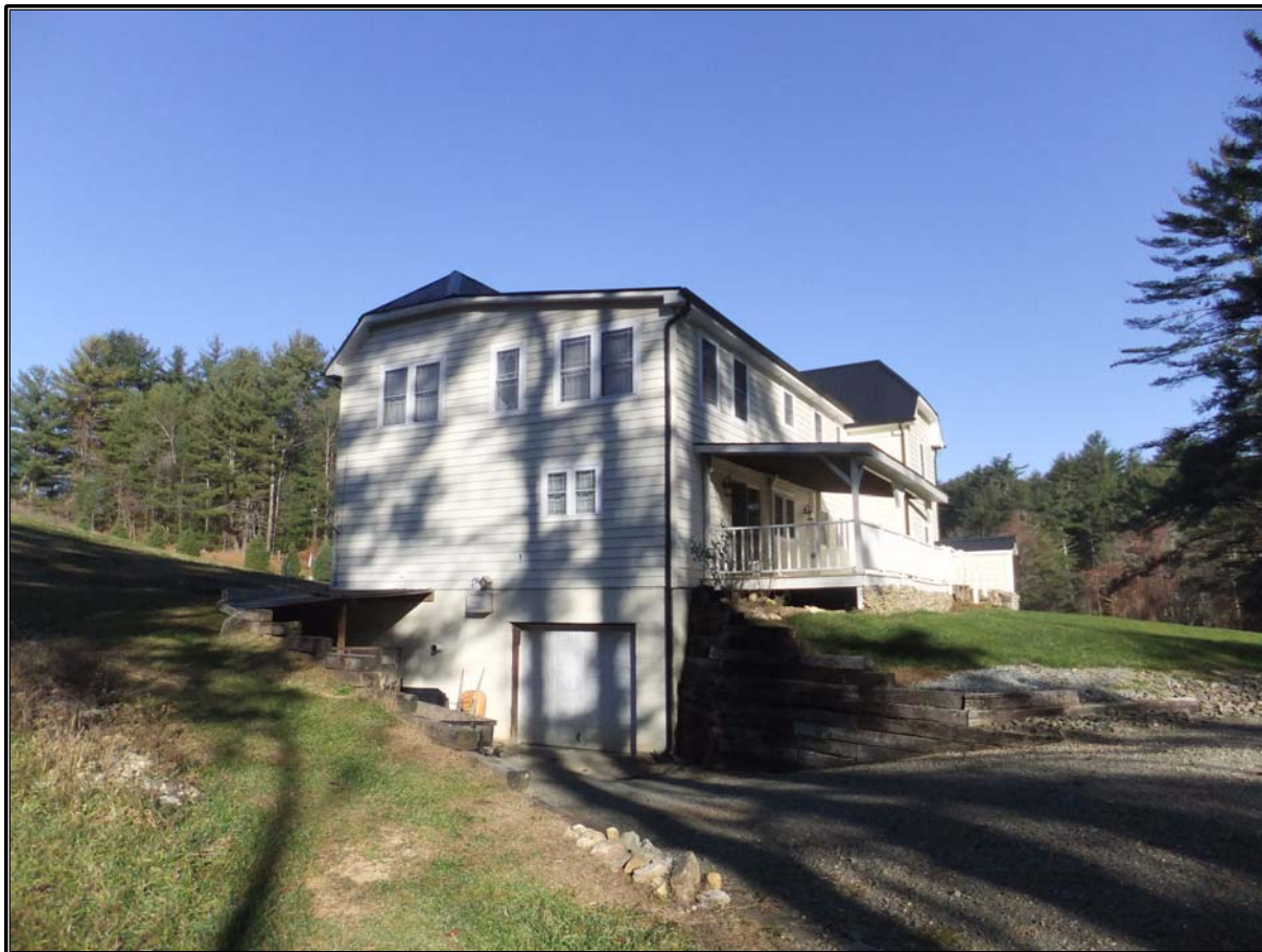
Figure 9. R.L. Hendrix House (AL 198): Northwesterly view of rear elevation.
