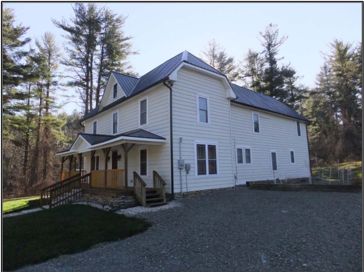
Figure 6. R.L. Hendrix House (AL 198): Southeasterly view of the residence.
